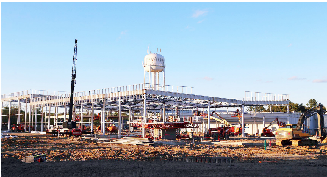
Saint-Gobain Performance Plastics facility construction.
