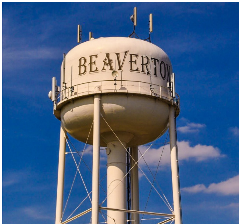
Beaverton water tower Source: City of Beaverton
